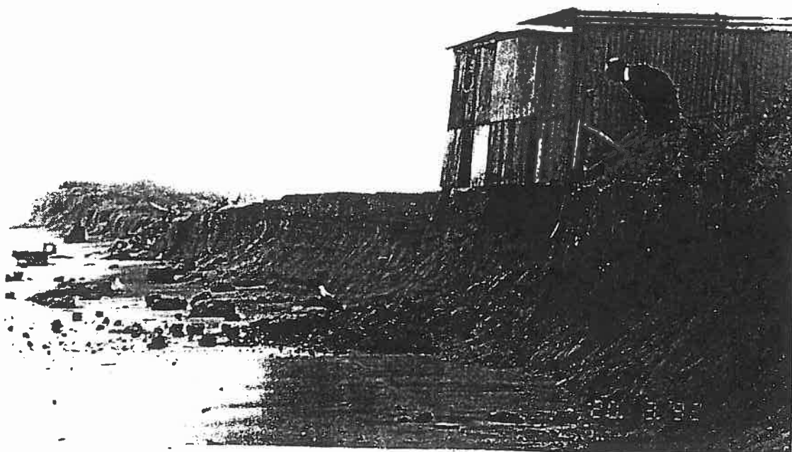
Photographs of Recent Coastal Erosion at Hokitika. (West Coast Regional Council Photographs 20.3.1992).
